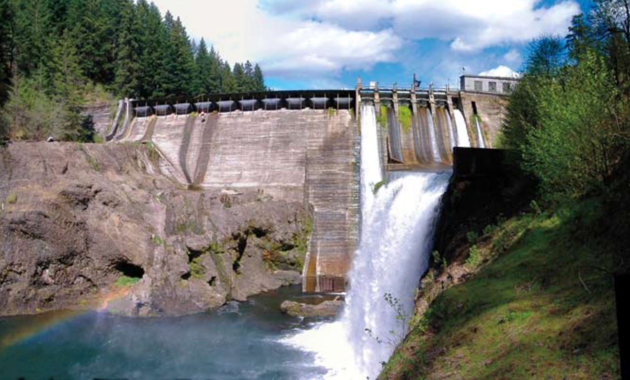
REMOVAL OF THE 125-FOOT-TALL Condit Dam (above) begins this fall. The century-old hydroelectric dam on the White Salmon River was built without fish ladders that would allow salmon and other species to migrate upstream. Removal of the dam will open up 33 miles of steelhead spawning habitat. Below, rafters float a natural stretch of the White Salmon.
